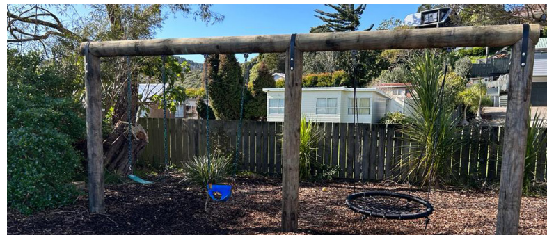
Early Childhood Swing Structure and Hangers with existing swing seats attached.
